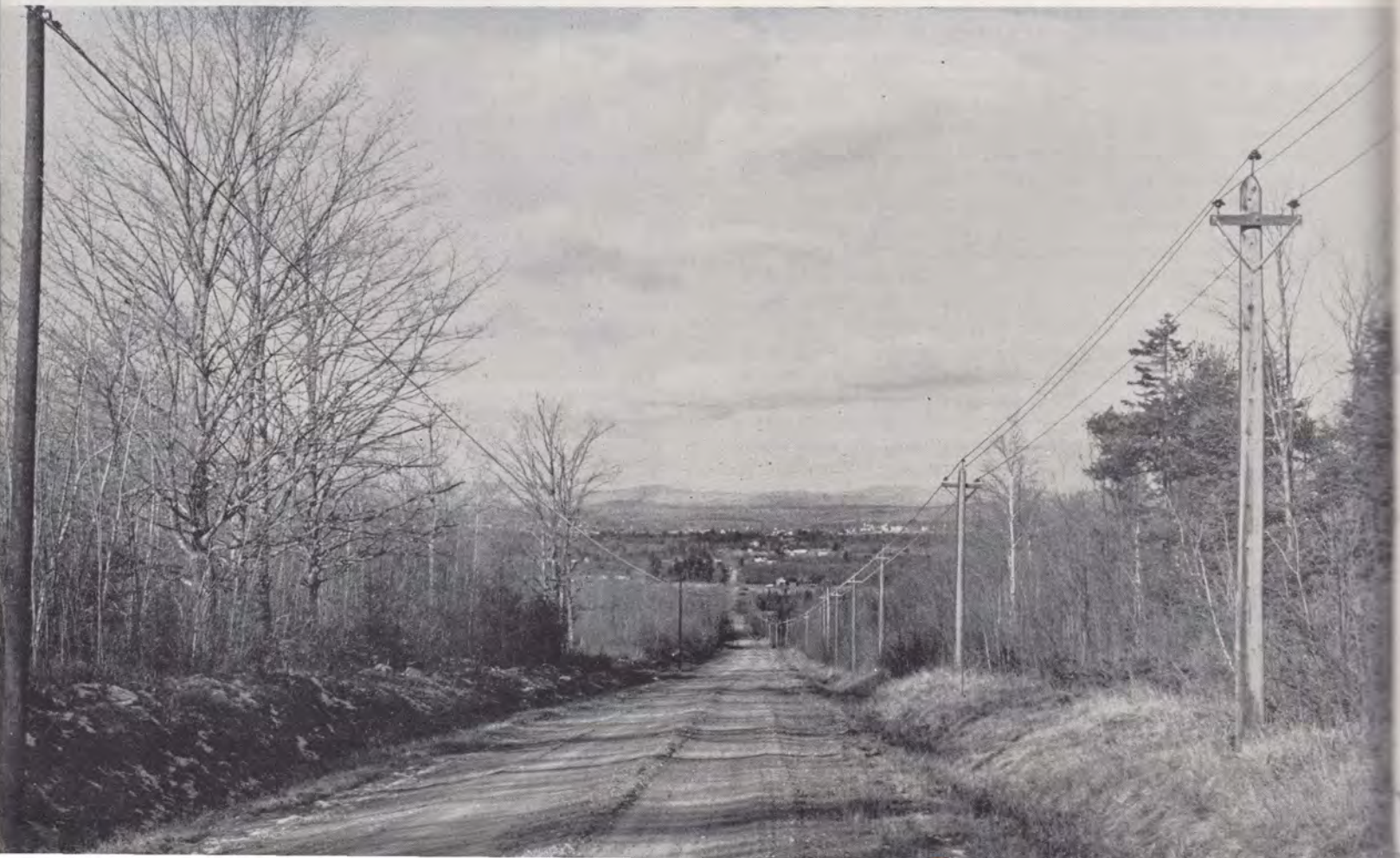
The picture below, taken in La Grange, Me., shows how new long-span construction (on the left) reduces number of poles.
