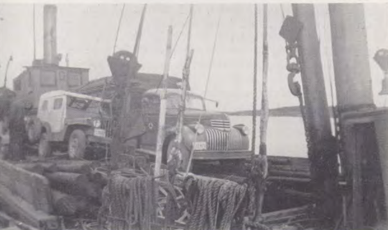
Destined for Northhaven and Vinalhaven was this sling-load of 26-25 and 30-foot poles being hoisted aboard the lighter.
