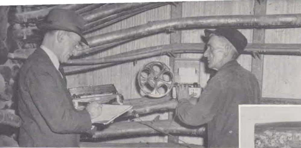
In the Liberty, Hancock, Hubbard cable vault at Harrison Avenue, Boston, Testers Edward V. Leonard and Charles Sullivan take readings.
