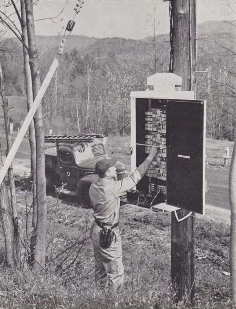
At the side of a road running between Bristol and Meredith, N. H., Harry Wood checks M-1 Carrier equipment.
