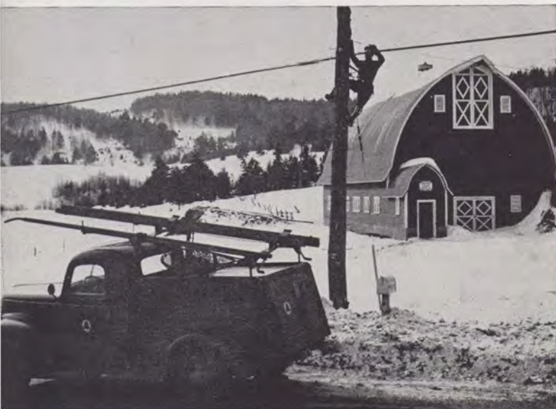
In winter weather Donald T. Fisher, Installer-Repairman, connects a line to a farmhouse in Morrisville, Vermont. Since the war about 50,000 new rural customers have been provided with telephone service—a 46 per cent increase.
