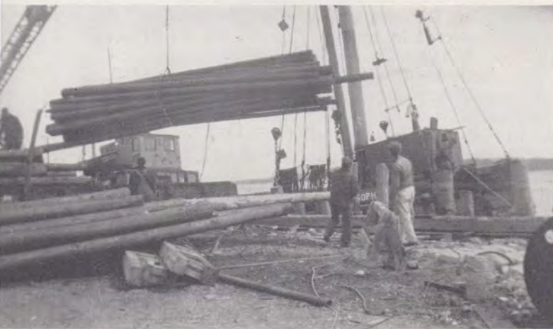
Destined for Northhaven and Vinalhaven was this sling-load of 26-25 and 30-foot poles being hoisted aboard the lighter.
