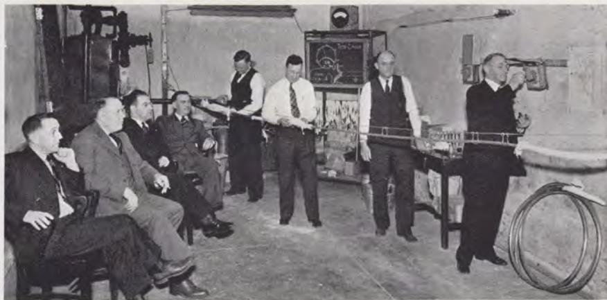
One of the classes recently held in Springfield on the use of desiccant in drying wires in cable. Left to right, William Langan, Wallace McInnis, John Beasley, Thomas Cane, Oliver White, James Logan, Myron Rogers, Instructor; and Edward McInnis shown repairing an open in No. 14 type terminal.
