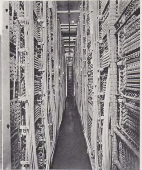
(Below) The new Diesel engine alternator equipment in the new Newton central office. (Right) Line link frames—Wiring aisle showing cable drawn in place prior to stripping and forming.
