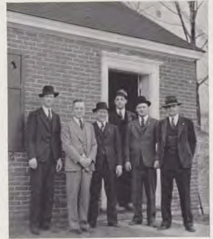
New Gorham Community Dial Central Office Building and group participating in conversion. Left to Right: George D. Bradstreet, Chief Switchman; Charles H. Anderson, Division Traffic Engineer; George J. Grafton, Switchman; Clyde B. Brooks, C. O. Inspector; Robert L. Gardenier, Recon. Foreman; Albion K. Wallace, Service Foreman.
