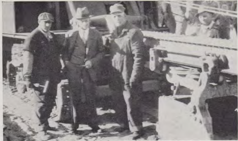
Arthur M. Warren, center in the above group, who worked with the Worcester Street department during a program of street improvement and thereby saved our equipment from being damaged by steamshovels, etc.
