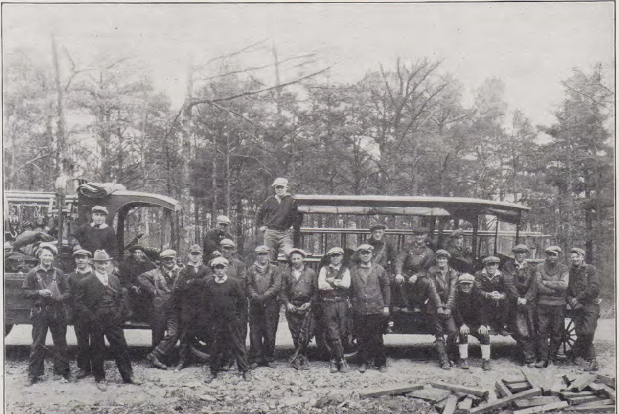
ON THE MIDDLEBORO-WAREHAM TOLL CABLE JOB—THE SETTING UP AND PULLING IN CREWS FROM NEW BEDFORD
