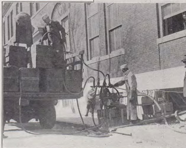
THE NEW MOTOR-DRIVEN ACID PUMP IN ACTION ON THE HIGHLANDS JOB
