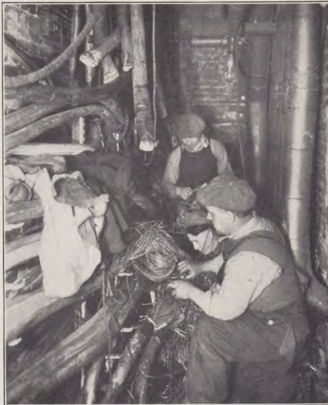
CUTTING OUT THE OLD—CUTTING IN THE NEW
