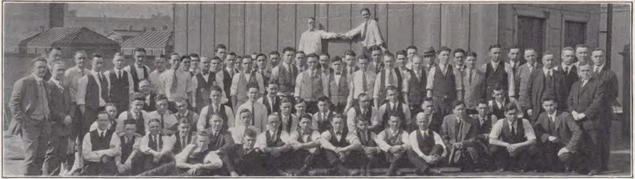
PART OF EQUIPMENT INSTALLATION FORCE
