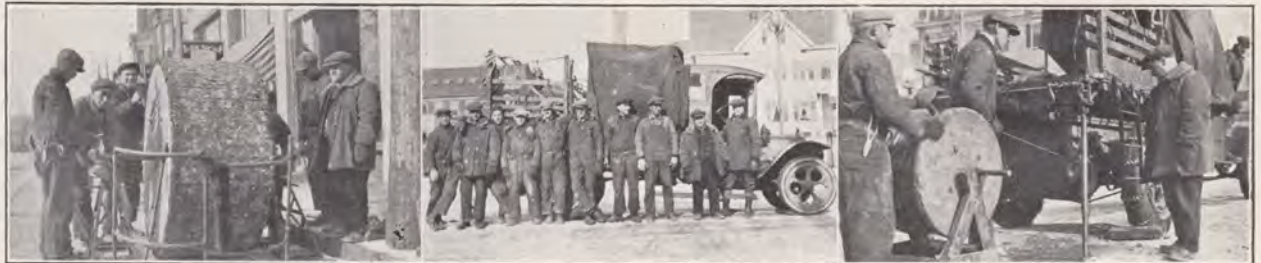
JIM WILKINSON'S GANG ON THE JOB AT BROCKTON
