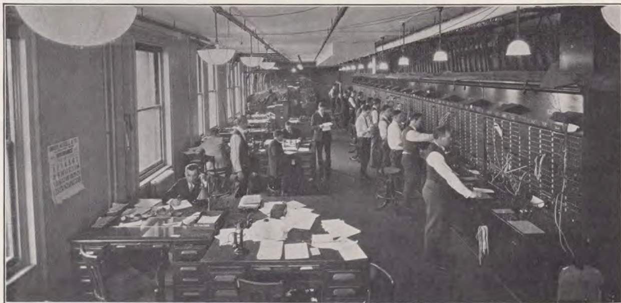
TESTING LINES AS CUT IN ON NEW TEST BOARD
