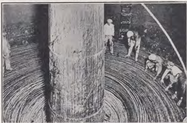
Coiling cable in one of the cable tanks aboard the Bellwood
