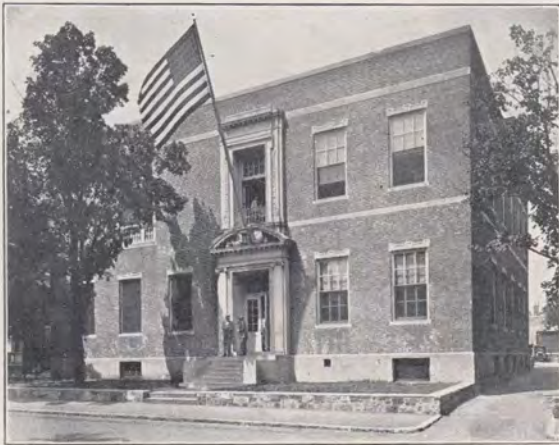
ASPINWALL CENTRAL OFFICE
