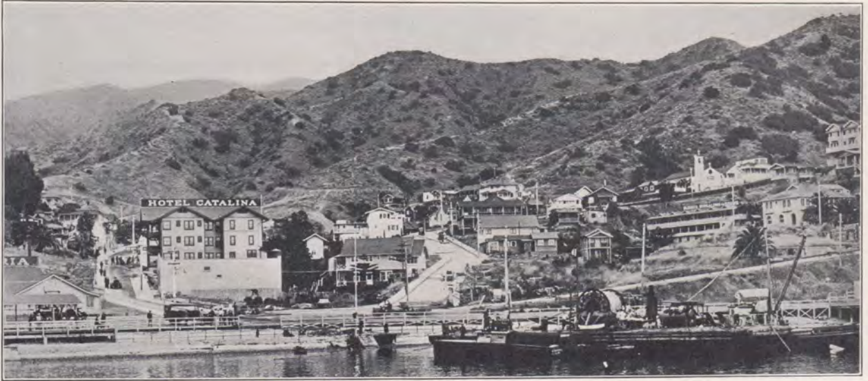
Pulling in the shore end of the east cable at Avalon from the barge. The central office is just beyond the Hotel Catalina
