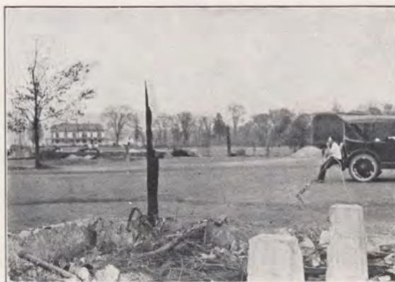
WHAT WAS LEFT OF 10 SECTIONS OF TOLL SECTION 110
