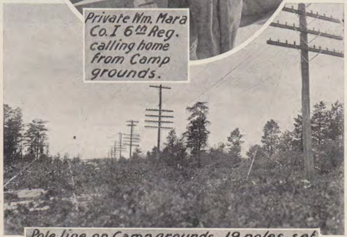
Pole line on Camp grounds, 19 poles set in one day.
