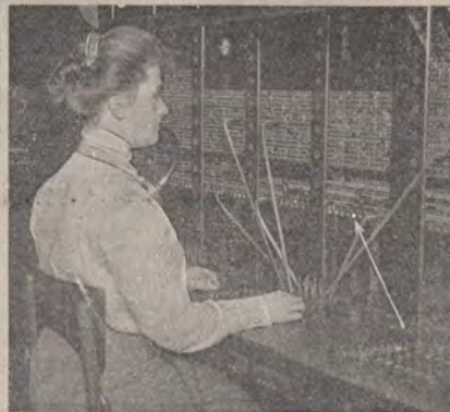
The operator is sitting, at attention, when a light glows in the panel in front of her. She can connect a caller with any subscriber in that exchange, but she is assigned to respond to the calls of only a limited number of subscribers whose signals are these lights showing at her particular position. The arrow indicates the light.
