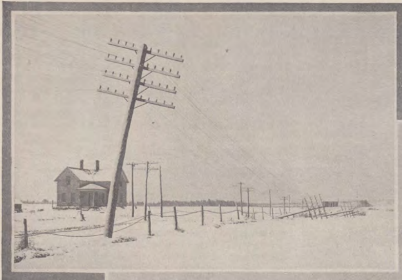
Showing Long Stretch of Wires Laid Flat
