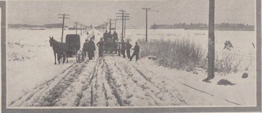
Putting up Emergency Cable
