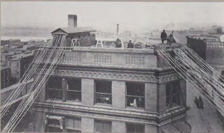
This was the telephone exchange in Kansas City, Mo. in 1895, when WE installers were putting in a new exchange. All wires still came in over the rooftops.
