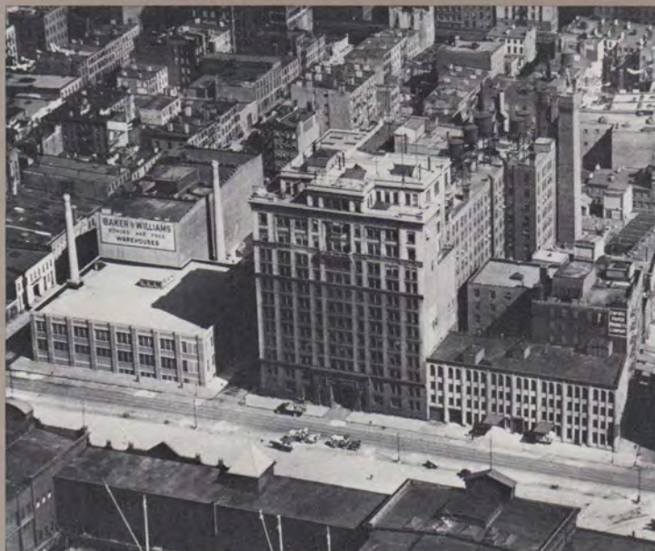
Western Electric's engineering department spawned Bell Labs in 1925. Tall building in the center became the new company's home.
