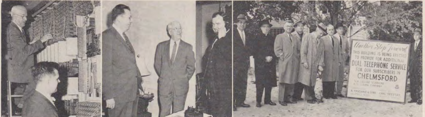
Left: This photo was taken just a few seconds before the shims were pulled in the new Dial Central Office at North Chelmsford. Center: Mr. McAndrews, member of the Board of Selectmen, places the first call from the ALpine 1 Central Office. Louis M. Reder, Manager, and
