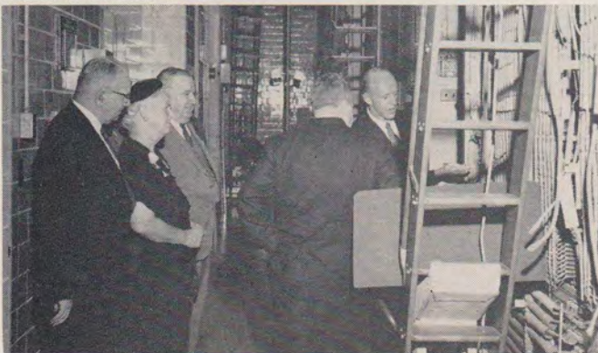
Mr. Barney and this group listen as John A. Bosanquet, Central Office Switchman, shows them the complicated mechanism in a New England Company equipment room.
