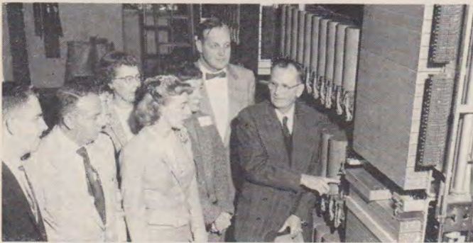
These teachers listen intently to Francis E. McKeon, Central Office Supervising Switchman, who is speaking on the operation of the central office equipment.
