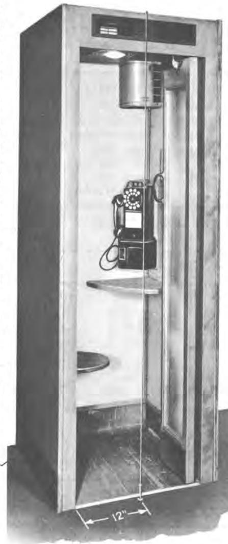
Fig. 2 - 11-type Booth with Plumb Line
