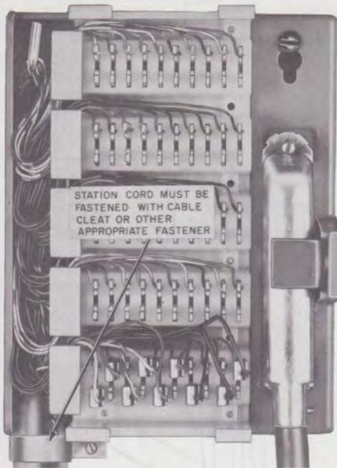
(ABOVE) TYPICAL INSTALLATION OF 161A ADAPTERS ON 66E TYPE CONNECTING BLOCK.
