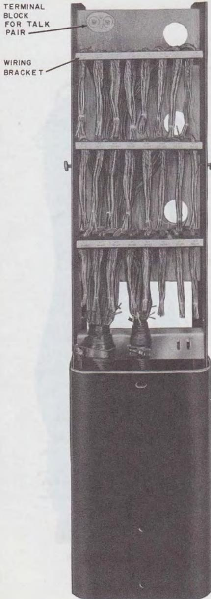
*cable pair is available, use cross-connecting wire for piecing out. Do not substitute an odd-colored wire.*
