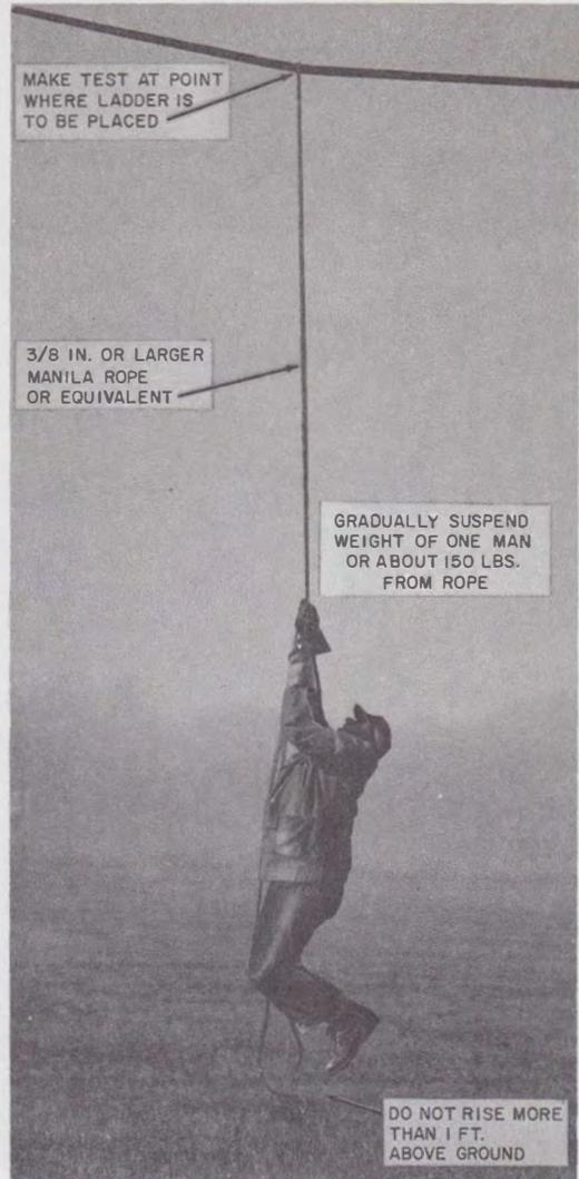
**Fig. 2—Testing Strand Prior to Placing Ladder**
