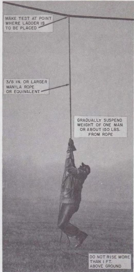
**Fig. 2—Testing Strand Prior to Placing Ladder**
