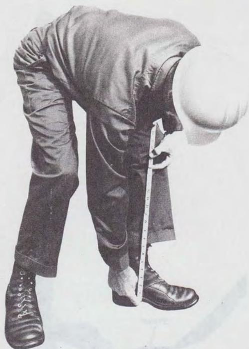
Fig. 8—Measuring for Climber Length
