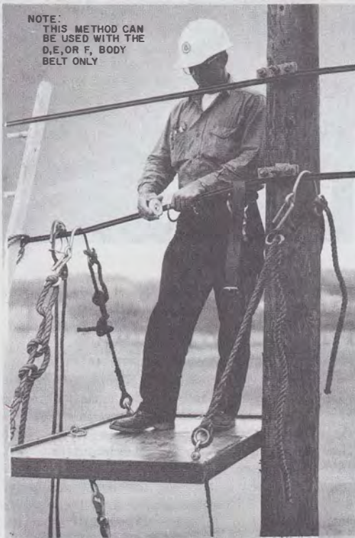
Fig. 6—Method of Using D, E, or F Body Belt With Safety Strap
