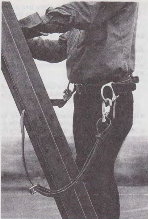
Fig. 4—Method of Using Safety Strap When Working From Ladder
