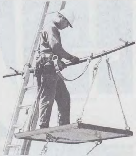
Fig. 7—Method of Using Safety Strap When Using Other Than a D, E, or F Belt
