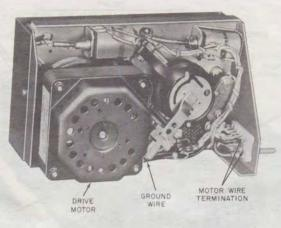
Fig. 5-KS-19245, List 2 Recorder, Motor Side
