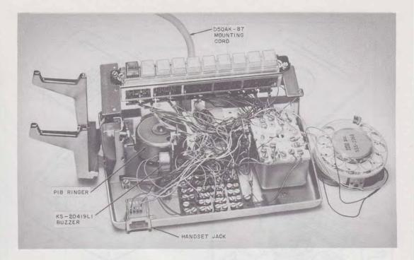
Fig. 4\_\$30CT (MD) Telephone Set Base, Dial Removed\$
