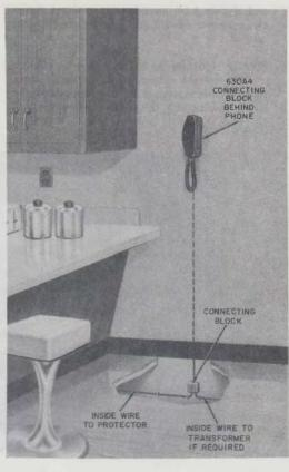
Fig. 3—♦Typical Installation of a Wall TRIMLINE
