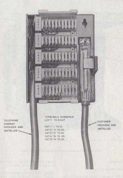
Fig. 3—66E3-25 Interface Connecting Block (Optional)
