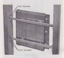
Fig. 12—113D Apparatus Box, Typical Installation (Rear View)
