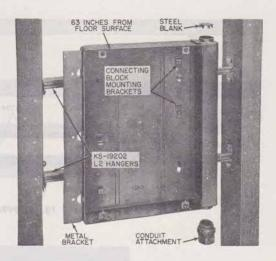
Fig. 11—113D Apparatus Box, Typical Installation (Front View)
