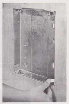
Fig. 15—113E Apparatus Box, Showing Installation Fig. 16—113E Apparatus Box, Showing Installed D-179941 Kit of Parts
