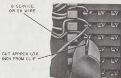
Fig. 7-Cutting B Service or SK Station Wire
