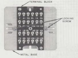
Fig. 4-149A (MD) Adapter, Cover Removed
