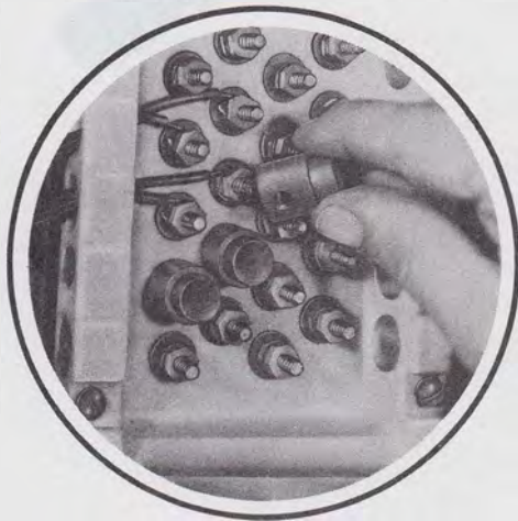
Fig. 19—Installing Binding Post Caps
