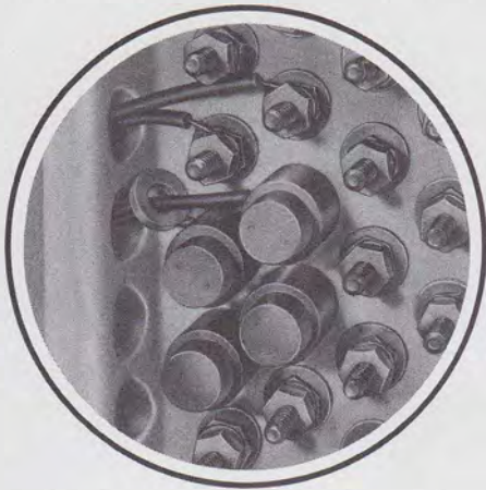
Fig. 20—Installed Binding Post Caps with KS-6660 Indicator
