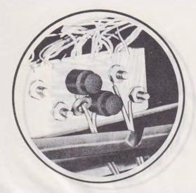
E binding post caps and indicators used with 49A cable terminal.
